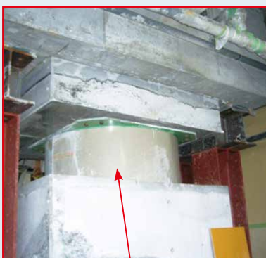
Seismic isolator
