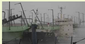
Collision of a tanker into the connection bridge of the Kansai International Airport
