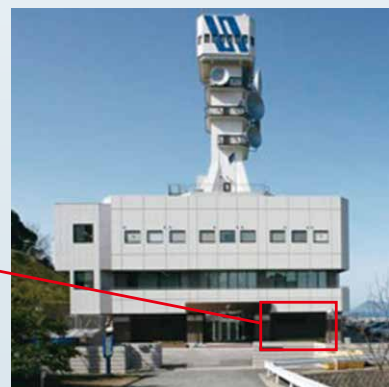
Antiseismic reinforcement at a Vessel Traffic Services Center
